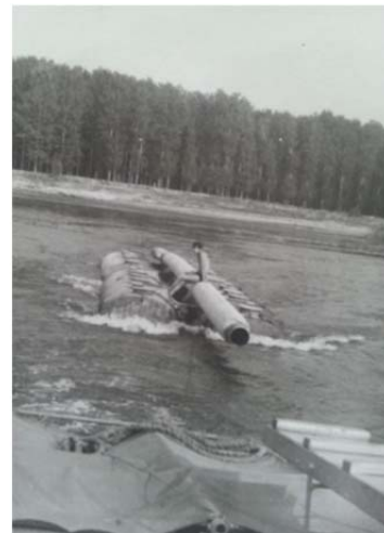
Photo 3. Mount on the bottom of the pipe.
