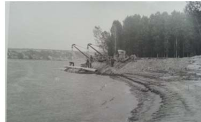
Photo 2. Oil Pipeline Install.
