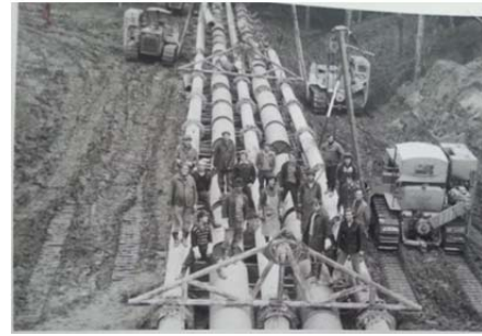
Photo 1. Danube crossing pipeline install.
