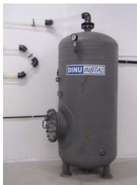
Fig. 5. Rezervor vacuumat vertical.
